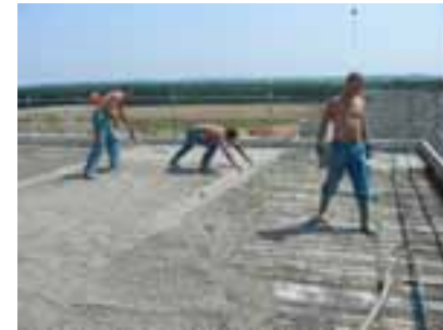
• Coulage dalle de compression
